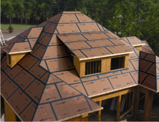
HERE IS A ZIP SYSTEM "ORANGE" ROOF
